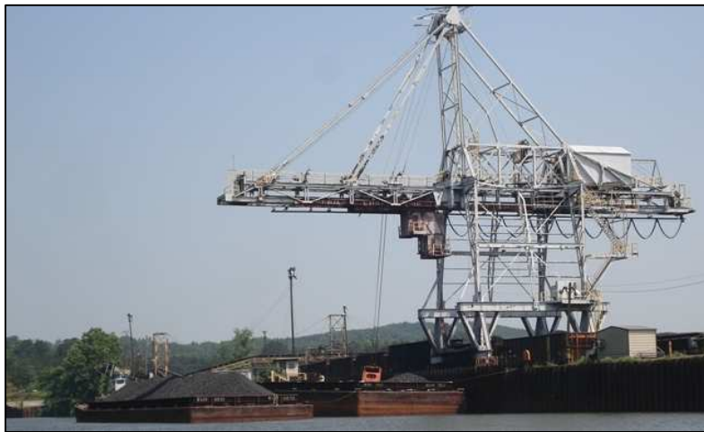
Figure 7: River view of Birmingham during "marine recon mission" with the wonderful old 1920's era overhead crane - well worth modeling.
